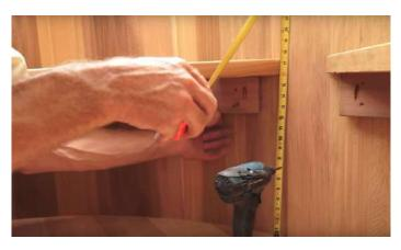
Measuring 17 1/2" from the floor to the top of the bench on each end should make sure that the bench is level.
