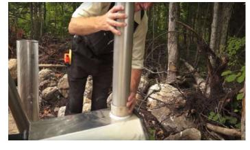
Slide the bottom stack pipe into the top of the heater.
