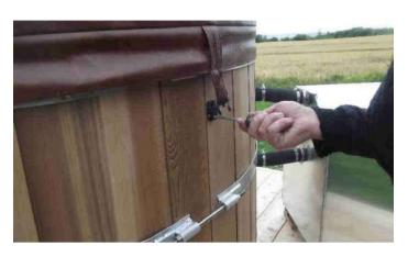
If you live in a high wind area, you will need to secure the cover so it doesn't blow off. This can be done by using the attached hold-down straps or by other means. To use the hold-down straps, let each hang down along the outside of the tub. Use a pencil and mark the bottom of each buckle on the side of the tub. Next separate the buckle (two parts) and screw the bottom part to the side of the tub at your mark with small (1") stainless steel screws (included).
