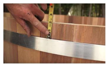
Using the same method as the bottom band, measure 2" from the edge of the top staves to the top of band.
