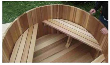
By trial and error, position the three assembled benches into the hot tub spacing them equally apart.
