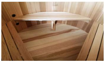
The Cedar Hot Tub has 3 benches. They each sit on two end brackets attached to the walls, and one support in the middle attached to the floor.
