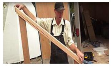
Make sure the bottom edge of the top railing is flush on the ends to the bottom railing and secure up through the bottom railing using 2" screws.
