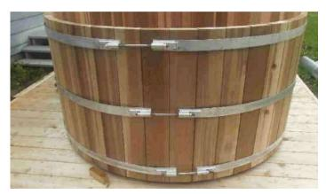
Assemble the other bands, and slip them into place with their tightening hardware rotated so that it is offset from the one below as shown. Snug them up as before just enough so that they won't slide out of position.
