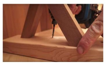
Fasten the bench supports to the tub floor using 2 1/2" screws.
