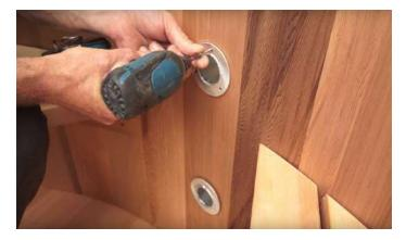
Put a bead of silicone caulking under the flange of the heater hose fitting, and fasten it with three supplied mounting screws as shown.
