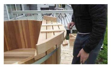
Make sure that the bench brackets are flush with the ends, and about ¾" back from the front edge of the benches.
