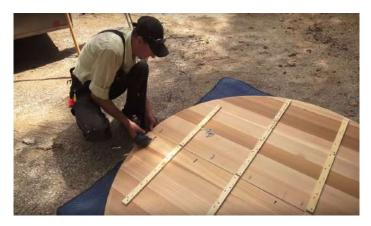
Line up the 2 pieces so the edges are flush, insert a 2 1/2" Kreg screw into the edges on both sides of the floor seam.
