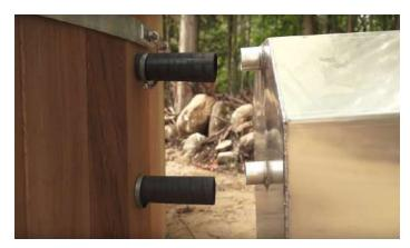
Slide the heater hoses onto the outer side of the heater hose fittings and secure with gear clamps.
