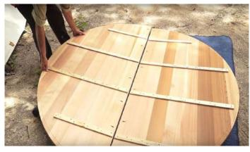
To protect the wood during installation, lay the 2 floor pieces upside-down on something soft like a blanket.
