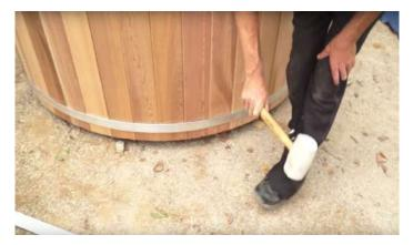
Work your way around the tub, hitting each stave with a firm tap on the bottom band.
