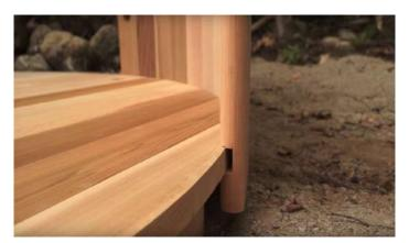
Leave a space between the edge of the floor and the bottom of the dado. Use the pencil line circle on the floor as a guide.
