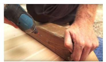
Using 3" screws, secure the joists to the floor as shown.
