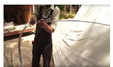
Locate the three stainless steel threaded rods and nuts for tightening the straps.
