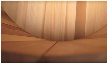
You must avoid having the floor seam line up directly with any of the seams between the staves.
