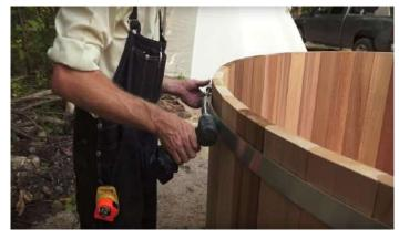
Tighten each band a little at a time, starting with the bottom band.
