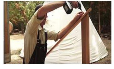
Center the bottom piece of the railing on to the railing supports and secure with 2" screws.
