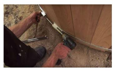
Tighten the nuts with a 3/4" wrench until the band is just snug enough so that it will stay in place.
