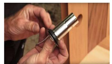
Slip the drain in place with the rubber gasket on the top side (inside the tub) and tighten the large nut underneath hand tight.
