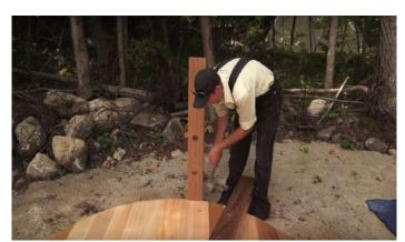
Start placing the staves with the dado (groove) over the edge of the floor as shown.
